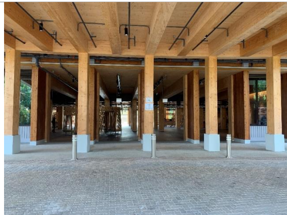
Gaia drop-off point
